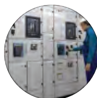
Pre- Commissioning & Testing
